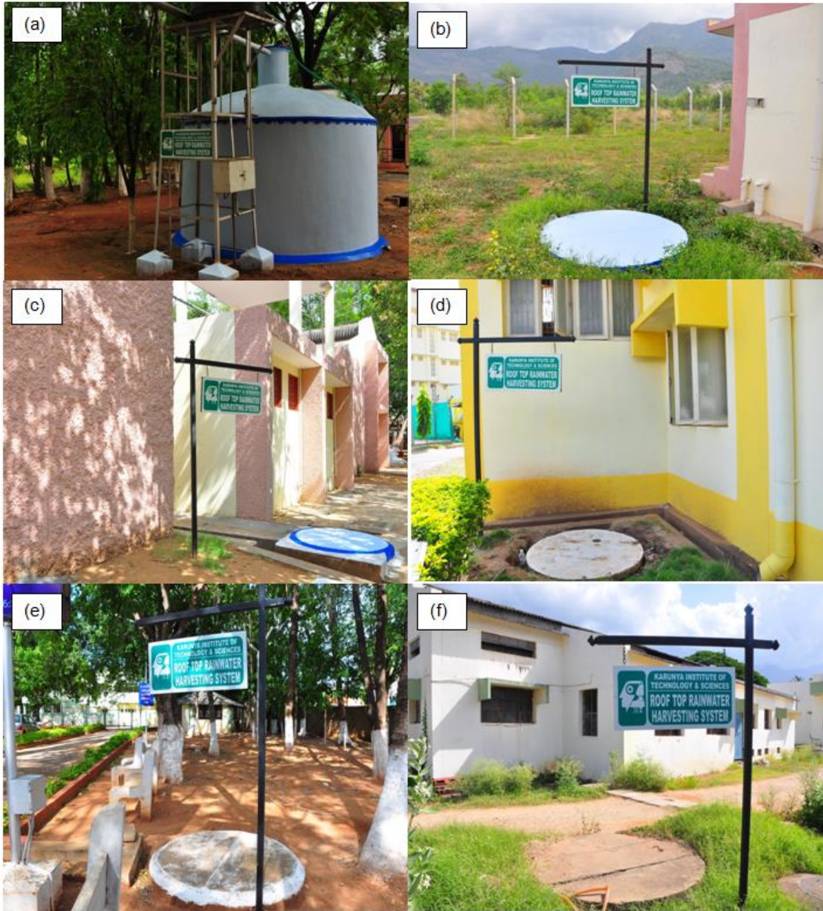
Soak pits located at (a) Administrative block (b) Aero space lab (c) Civil lab (d) Guest house (e) Hepzibah hostel and (f) Father Duraisamy Residence hostel
